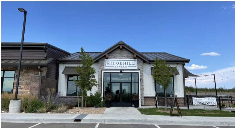
South Hill Subdivision 9th Filing - Windsor Apex Condominiums (Ridgehill Tavern)
